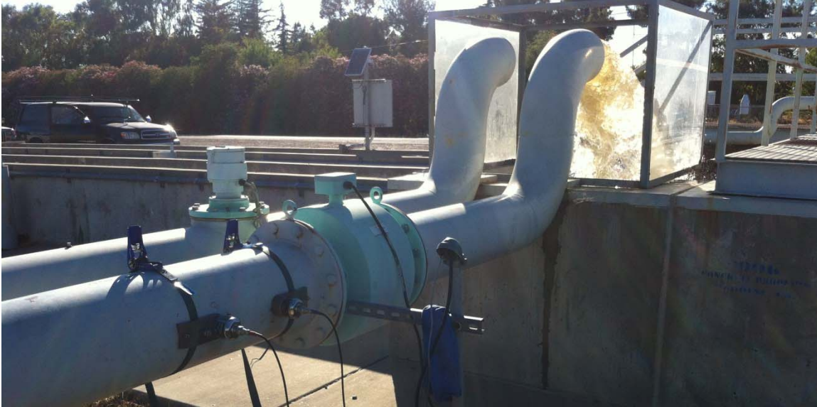
Figure 7. Water Specialties Magnetic Flow Meter at CSUC ATRC
