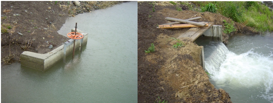
Figure 1. Standard Delivery Site Inlet (orifice gate) and Outlet (weir box)
